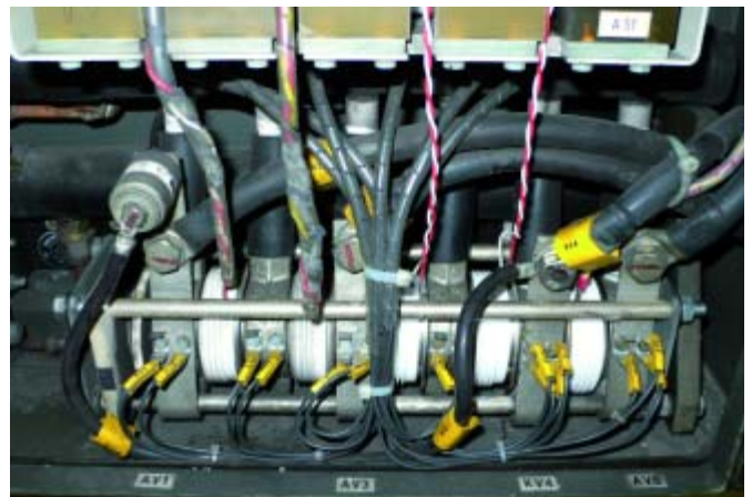
Figure 2: DC Chopper with RCT's before the conversion
