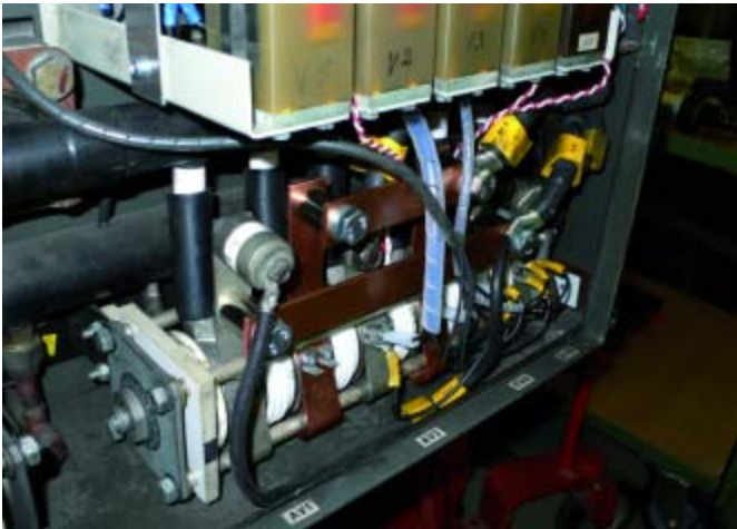
Figure 3: DC Copper converted with fast thyristors
