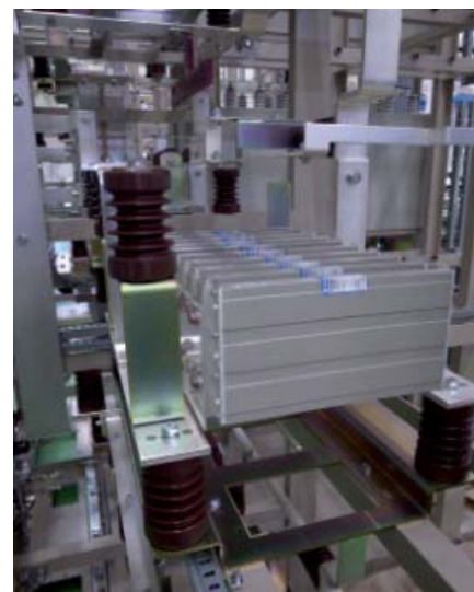
Figure 6: Fuses with low inductance for IGBT protection
