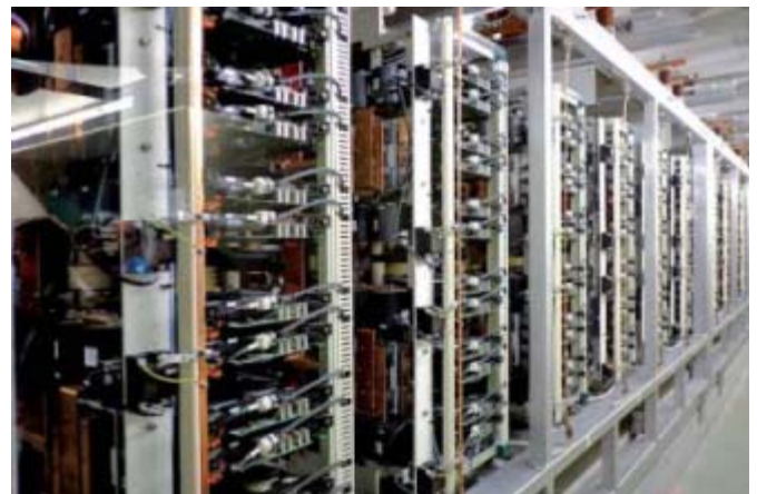
Figure 2: More than 1,000 IGCTs enable the pumped storage power plant Grimsel 2 to operate more flexible and efficient.
