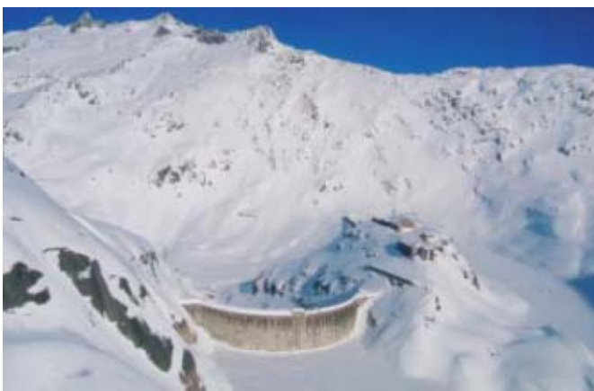
Figure 1: Hydro power site Grimsel in the Swiss Alps.
