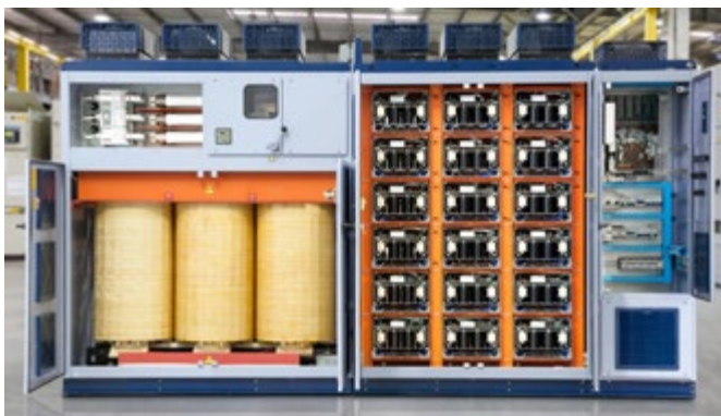
Figure 3a: MV3000 a 4160Vac 1500hp drive from WEG. Switchgear and transformer on the left and 18 cells (shown in detail in Figure 3b) in the center.
