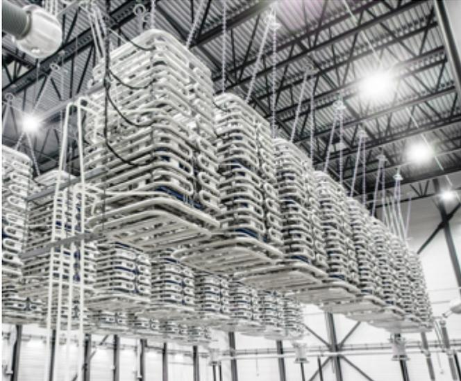
Figure 3: HVDC light valves
