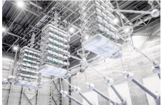
Figure 4: HVDC Classic valves from North East Agra multiterminal link in India
