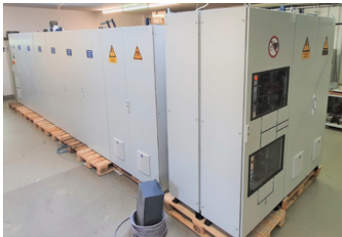
Figure 1: Not quite commonplace: the new 35kA surge current system of IPH in Berlin.
