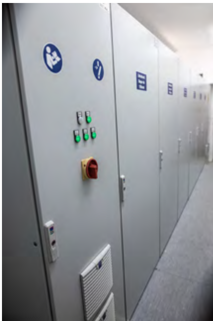
Figure 1: IRS Systementwicklung GmbH and GvA Leistungselektronik GmbH develop in close cooperation pulse power sources for up to 35kA.
