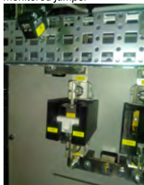
Figure 5: Current setting via resistance matrix and/or monitored jumper
