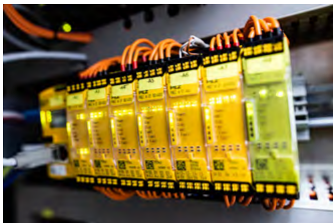
Figure 8: Safety control to avoid dangerous situations
