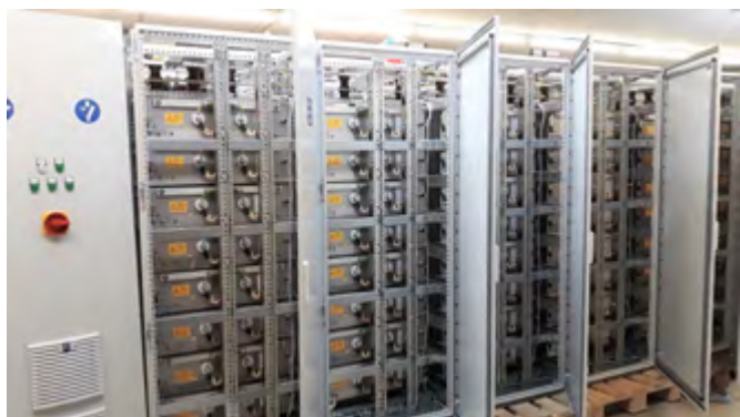
Figure 3: Huge capacitor banks from GvA buffer the necessary energy
